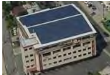
Installing solar PV system, PCKK, Palau Maldives
