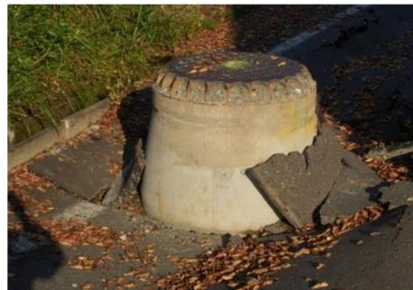
Protruding manhole due to soil liquefaction
