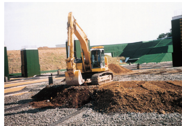
Covering the ash with soil following landfill
