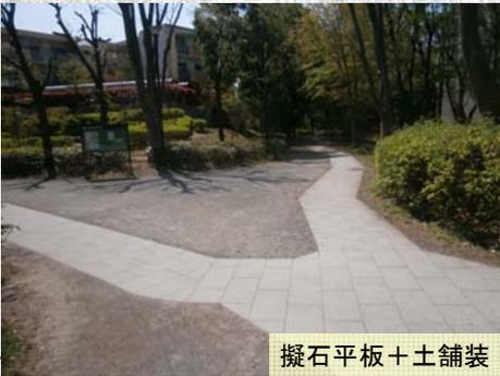
Photograph showing a paved path crossing a road, illustrating the '擬石平板+土舗装' (Artificial stone slab + soil paving) material used.
