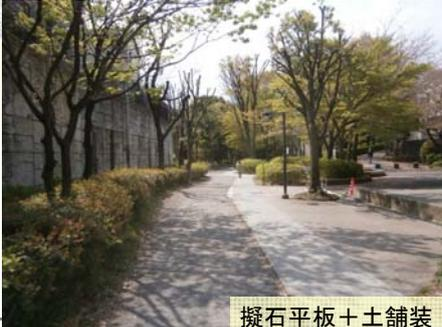
Photograph showing a paved path with trees and a building, illustrating the '擬石平板+土舗装' (Artificial stone slab + soil paving) material used.
